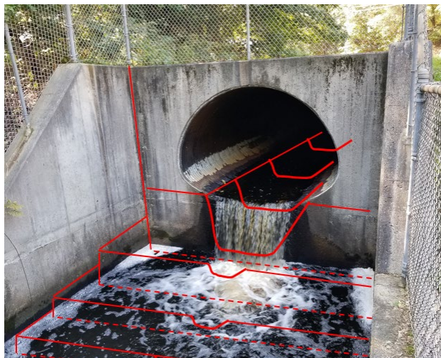
Figure 5: Alternative 6 View Shows the “Keyhole” Culvert exit
